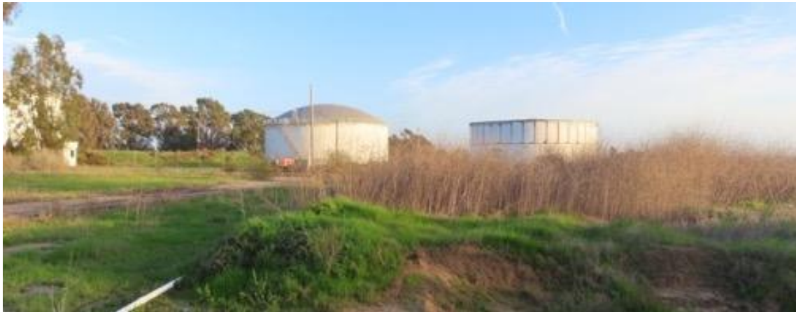
Fig 2: Elwood Marine Terminal restoration slated to start in Spring, 2024
